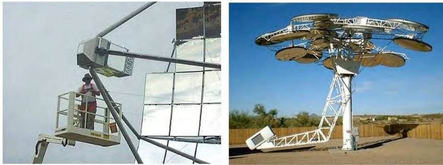
Figure 22.2 Accessing the solar receiver and Stirling Power Conversion unit for repairs and maintenance (WGAssociates, 2001).
