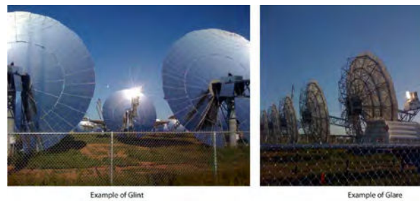
Figure 22.10 Glint and Glare can cause disturbance to motorists and airline pilots (Meyer, 2010).
