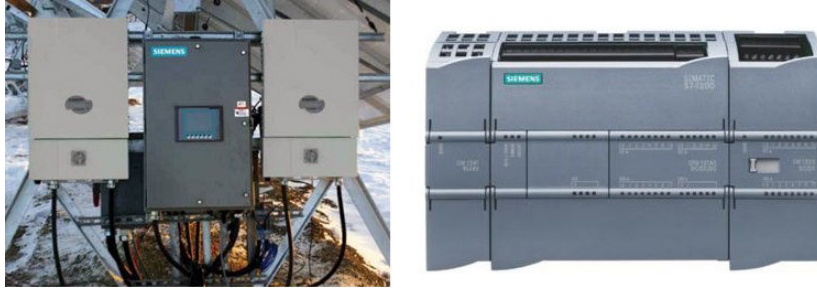
Figure 3: Trabant Solar Tracker controlled by Siemens Simatic S7-1200 controller with onboard Ethernet communication (?).
