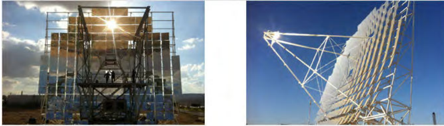
Figure 21.7 The HelioFocus concentrated solar dish with mirrors mounted on a flat surface (Smith and Cohn, 2010).
