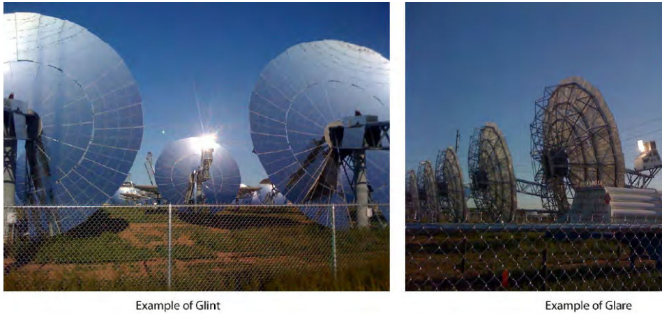
Figure 17.2 Examples to illustrate the hazards of Glint and Glare from concentrating solar power plants (Ho et al. , 2009)
