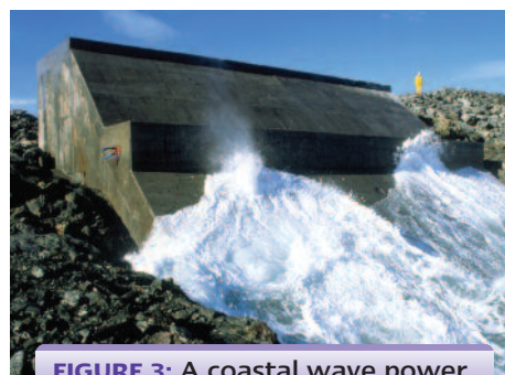
FIGURE 3: A coastal wave power station called 'Limpet 500'. It generates 500 kW of electricity, enough to power 300 homes.
