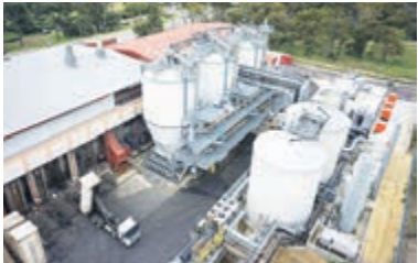
The DiCom plant in Shenton Park.
