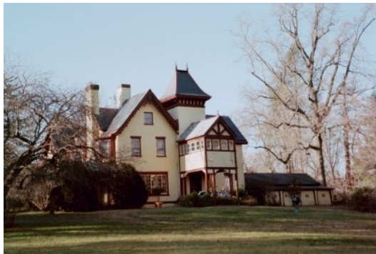
Figure 25: View of the Headley house from the east, including the main entrance. Harney's carriage entry-balcony has been turned into a sun room that relates to the rest of the house even more awkwardly. Photo by author, 2000.
