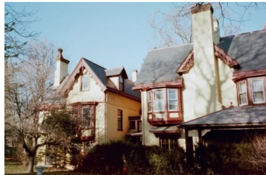
Figure 26: The south facade of the house has been greatly altered from the original, including the addition of a chimney through the gable and a large annex (1924), left, with different jigsaw ornamentation. Photo by author, 2000.
