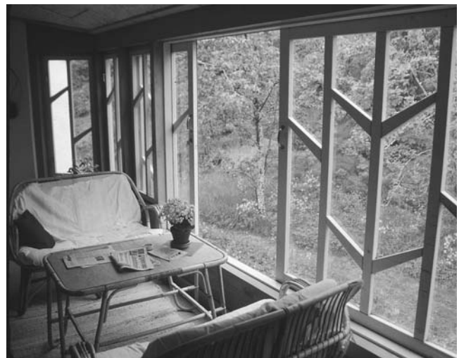
Balcony window wall opens for fresh air: This French balcony at the Vidar Clinic in Jarna, Sweden, when opened, connects this space to the surrounding landscape. Note the anthropomorphic mullion design and the low sill.
