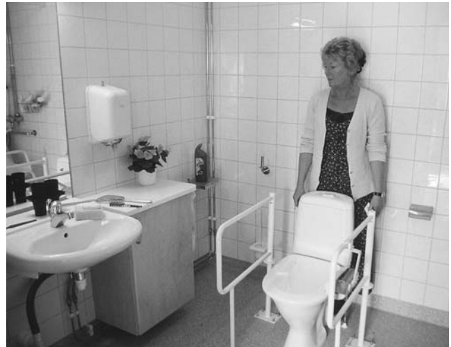
Toilet designs for accessibility vary: In the Kv Strykan project in Malmö, Sweden, space has been created behind the toilet to give caregivers more room to help residents who require two-person assistance.
