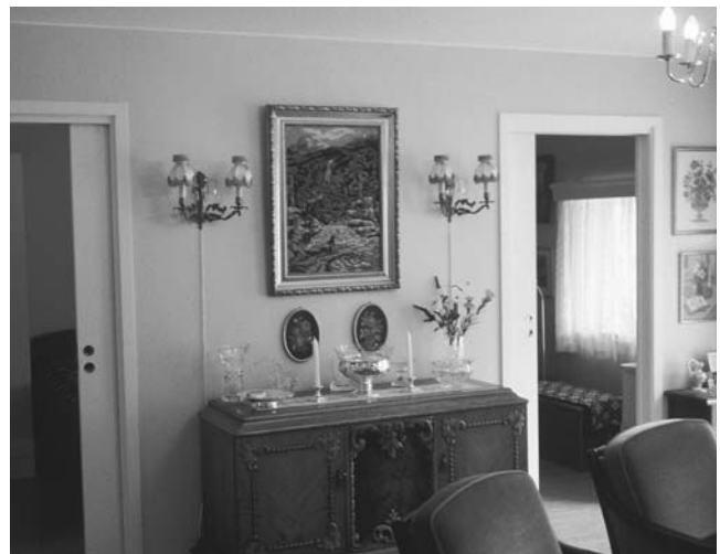
Two sliding pocket doors provide access: These two door in the Ensjetunet project in Oslo, Norway, link the bedroom with the living room but also allow caregivers to reach the bed from both sides, facilitating transfers.
