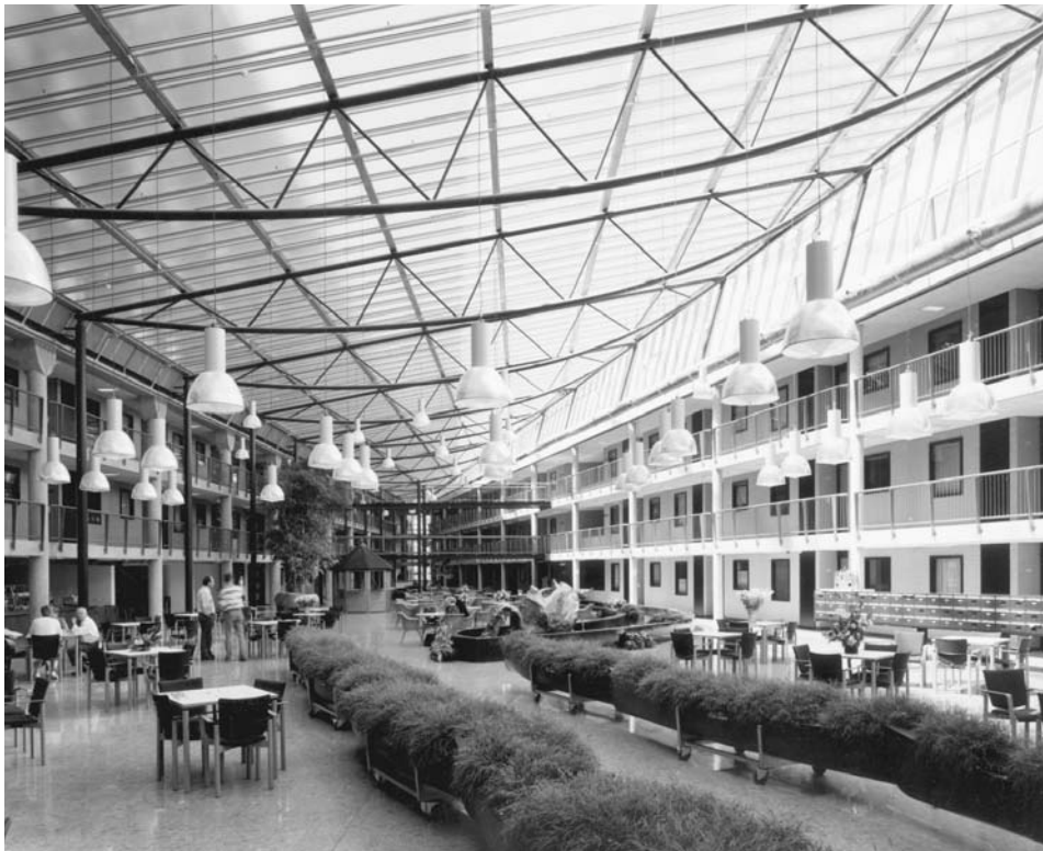
Central atrium is a public place: The atrium is a reverse bowstring truss structure covered by translucent glass. Landscape features, bridges, a restaurant, a soft-seating lounge, a koi pond, and a bistro bar are a part of this lively, light-filled space. (Photo: Marcel Van Kerckhoven)
