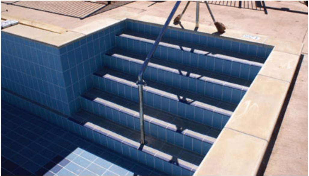
Figure A.11 Entry stairs with safety rail
