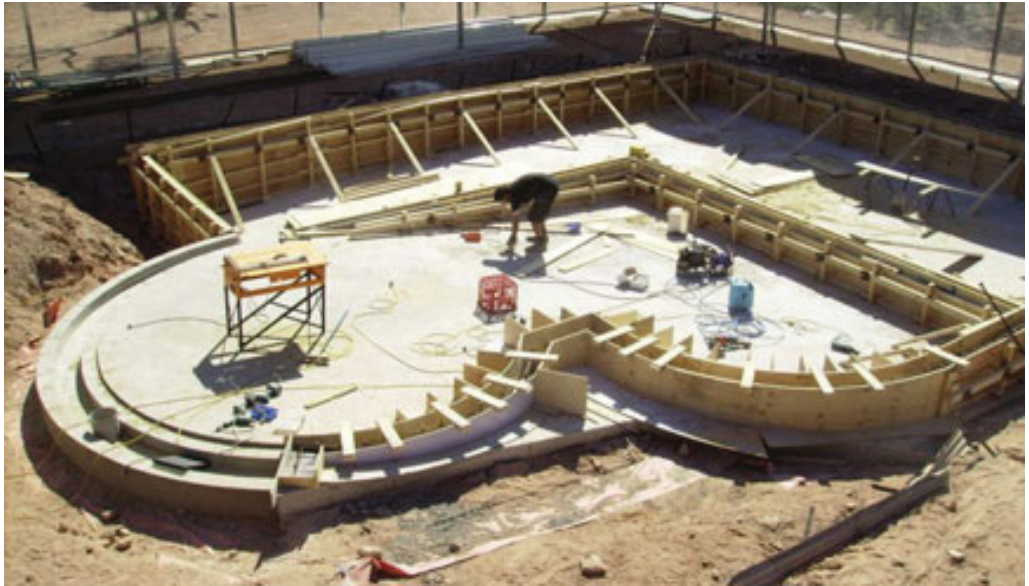
Figure A.2 Swimming pool under construction
