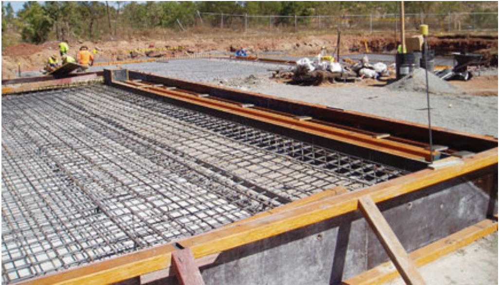
Figure A.8 Outdoor lap pool under construction
