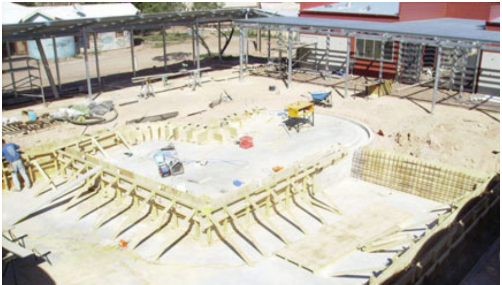
Figure A.3 Swimming facility under construction
