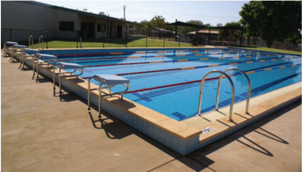
Figure A.10 Completed outdoor lap pool
