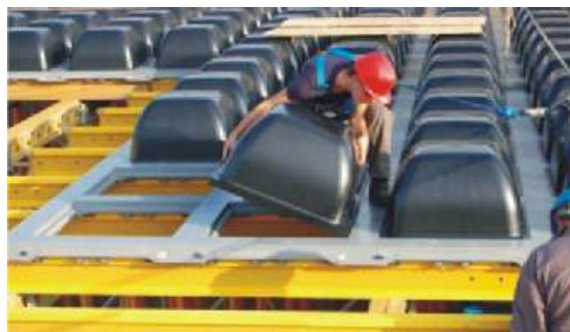
The light weight waffle slab formwork is more cost effective due to creation of void, which reduces significant volume of concrete consumed as compared to a solid slab. The slab is completely self supporting and does not require any special safety device or support platforms. The system can be assembled from below, providing additional safety for the job site workers.
