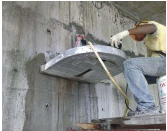
fect solution. Wire sawing is the newest cutting technique using diamond tools applied in construction works.
