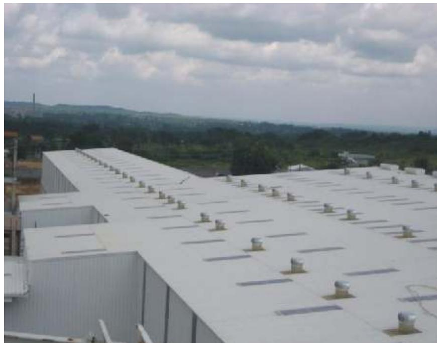
Interarch standing seam allows the customer to have a single piece panel covering the entire width of the building in lengths of upto 70m without breaks.
