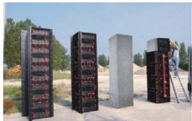
The first modular formwork meant for square and rectangular columns with 100 repetitions and with 105 different combinations of size and shape. Use of Geopanel star allows faster assembly due to light weight. The panels require less manpower in comparison to wood and steel formwork and can sustain 6200 kg per sq meter of concrete pressure. No releasing agent required after concrete pour and the material can be stored and stacked easily by just washing with water.
