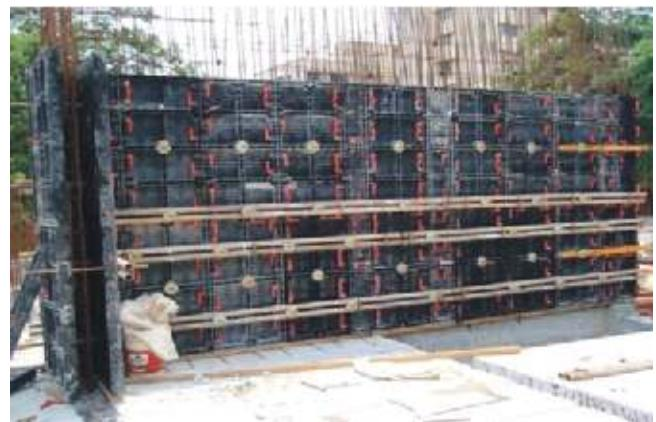
This is an easy and intuitive system of modular high resistive ABS plastic formwork for building concrete walls, basements, foundations and pillars lift walls etc. Compared to traditional wood or steel system, GEOPANEL® is more handy, cost effective and faster to assemble and dismantle. With different panel sizes, internal & outer corner elements can be used to form wall thickness from 100 mm to 400 mm.
