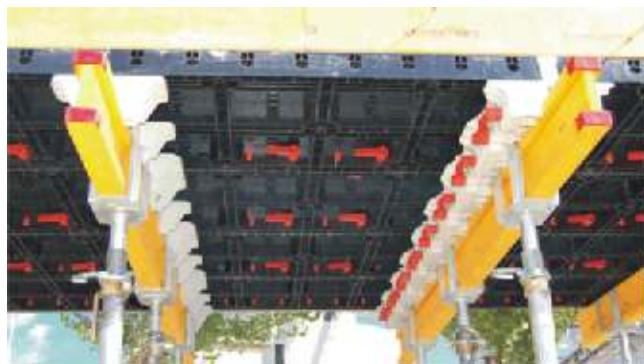
Geosky is an advanced high resistive ABS plastic formwork system for slabs. The combinations of main beam and sliding wedge can be used to make slab set up. The system can be dismantled very fast and reduces turnaround time of the slab system. With this system, partial removal of panel is possible within just one day. It is an ideal solution to pour any kind of slab, bidirectional, full or lightened.
