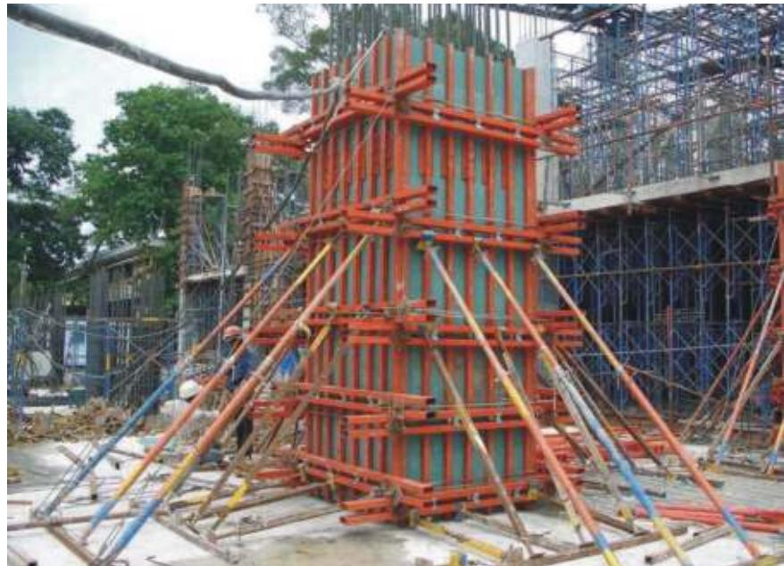
Providing much needed support: Systems formwork systems have come to the rescue of contractors helping them cut down on project costs and address the issue of labour shortage
