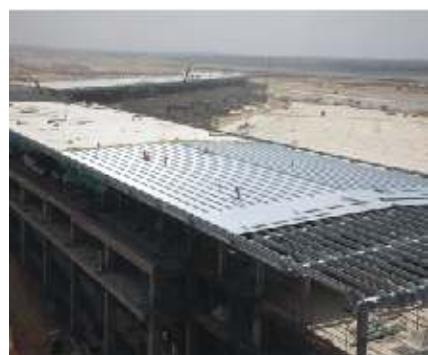
Tracdek metal roofing system for industrial and commercial buildings
