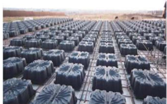
The advanced formwork system for voided biaxial slabs transforms full concrete in mesh of orthogonal beams. The advantages include weight reduction up to 40%, reduction of deformations, foundation load reduction and reduction of column width. The system is highly flexible and cost effective as it is possible to build spans of up to 20mtr. □
