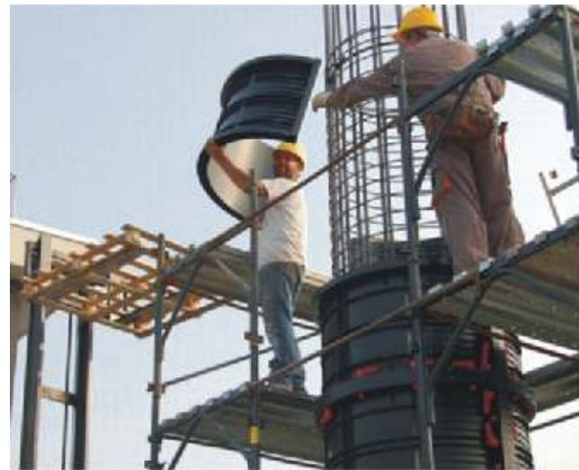
The first ABS plastic formwork customized for round columns with diameter ranging from 200mm to 1000mm. These panels can be reused up to 100 times. The concept is new and very different from wood and steel formwork. The use of panels allows faster assembly and removal al without releasing agent. The result is massive savings in manpower and shorter completion period for the project.
