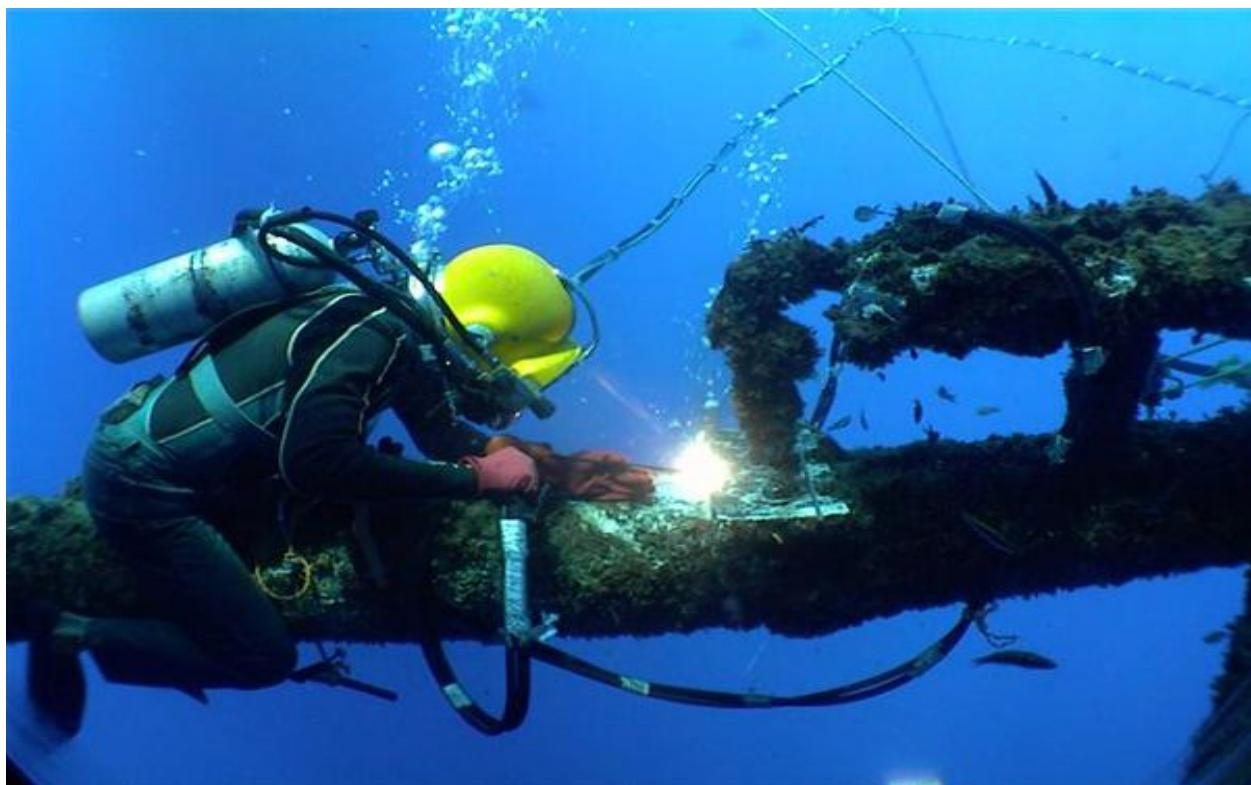
The increased freedom of movement makes wet welding the most effective, efficient and economical method.
