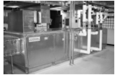
The general-service air-handling system used for the tests. It serves the classrooms, offices, and common areas of the Energy Resource Station with a nominal capacity of 7,800 cfm.
